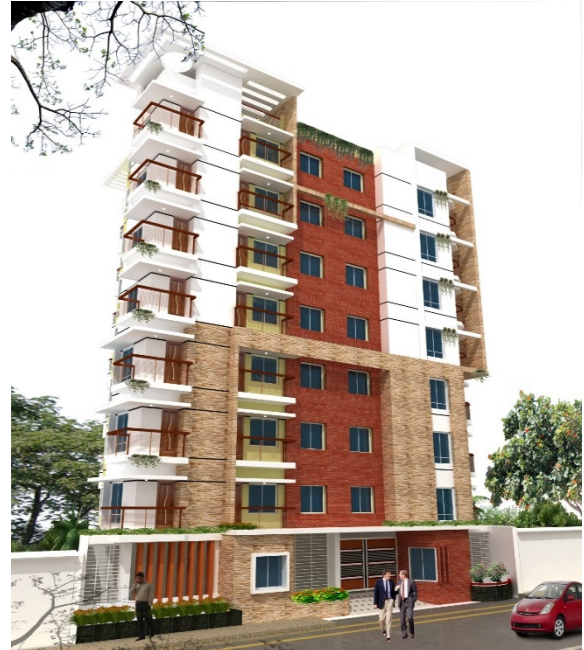
Client: Soiltech Ltd 08- (Eight) Storied Residential Building, Turag, Dhaka.
